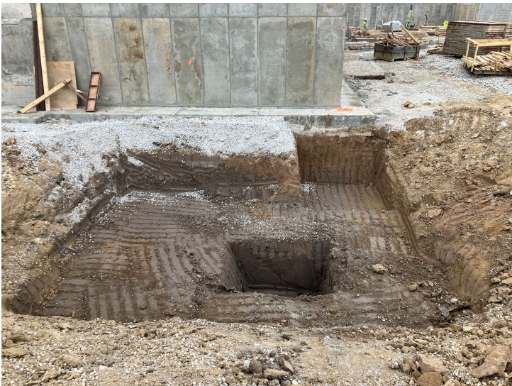
Elevator pit in building C
