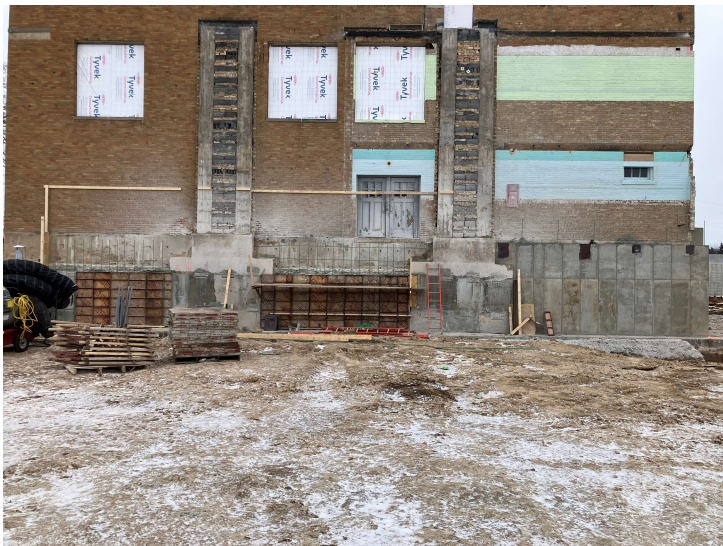
One-sided wall on Southend of building A
