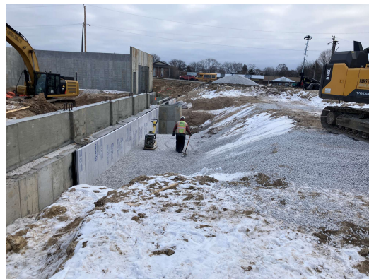
Stone compacting South end of building B
