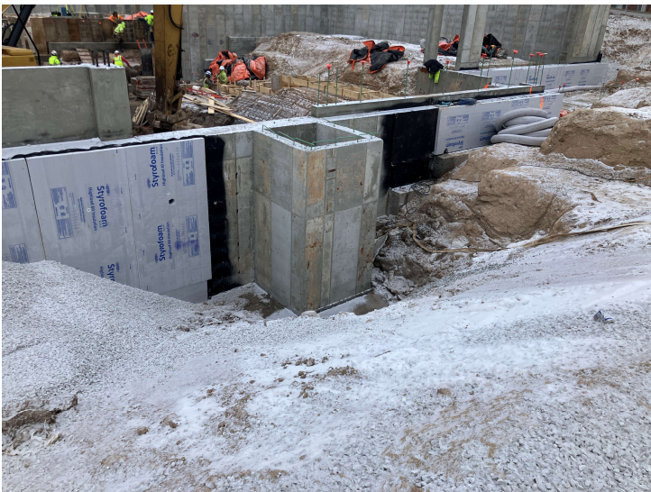
Water proofing southside of building B
