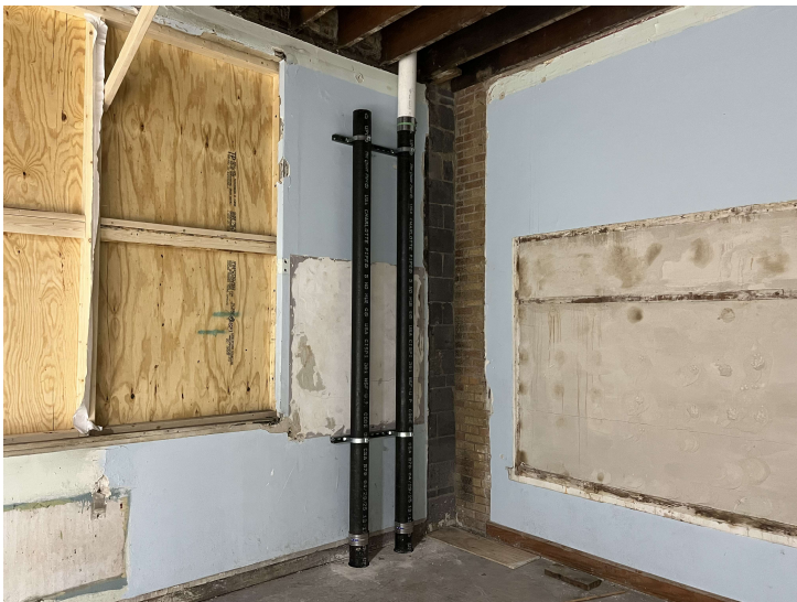
Building A roof conductor install
