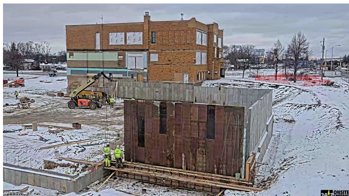
Southside of Building B wall forming
