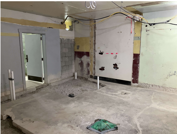
Backfill of underground plumbing after passed inspection
