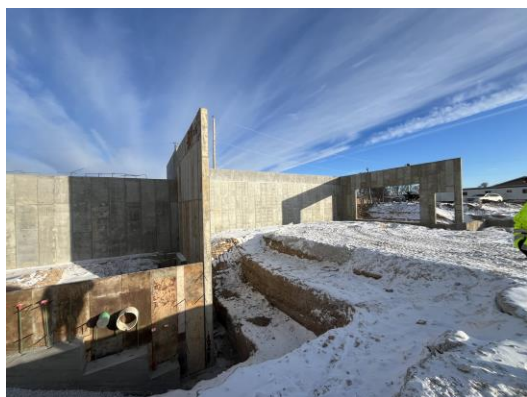
Southeast side of Building B wall forming
