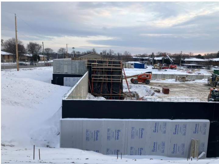
Waterproofing foundation walls on East side of Building B
