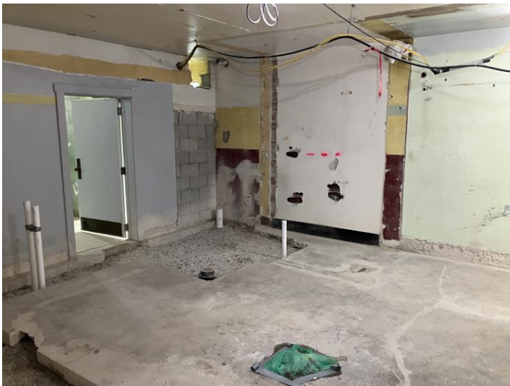
Backfill of underground plumbing after passed inspection
