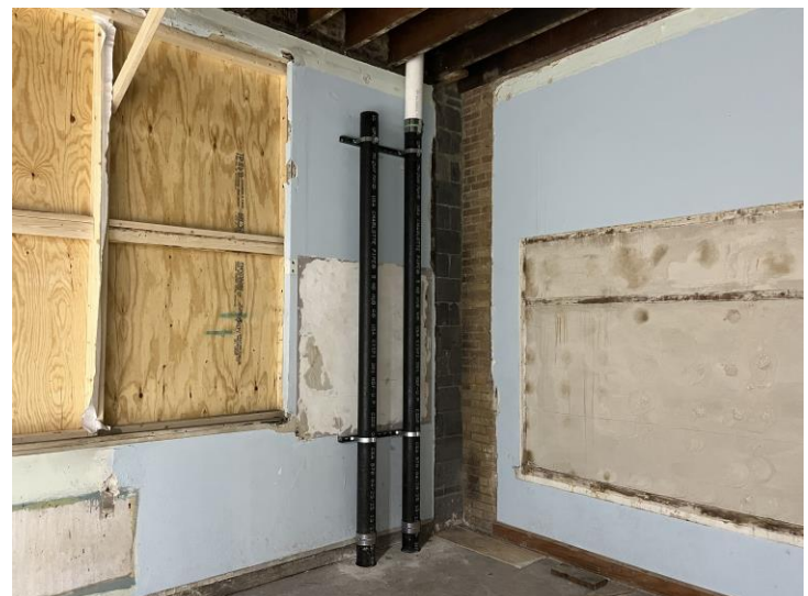
Building A roof conductor install
