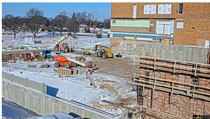
Southside of Building B wall forming
