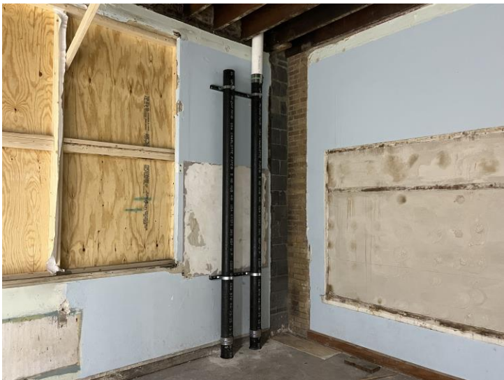
Building A roof conductor install
