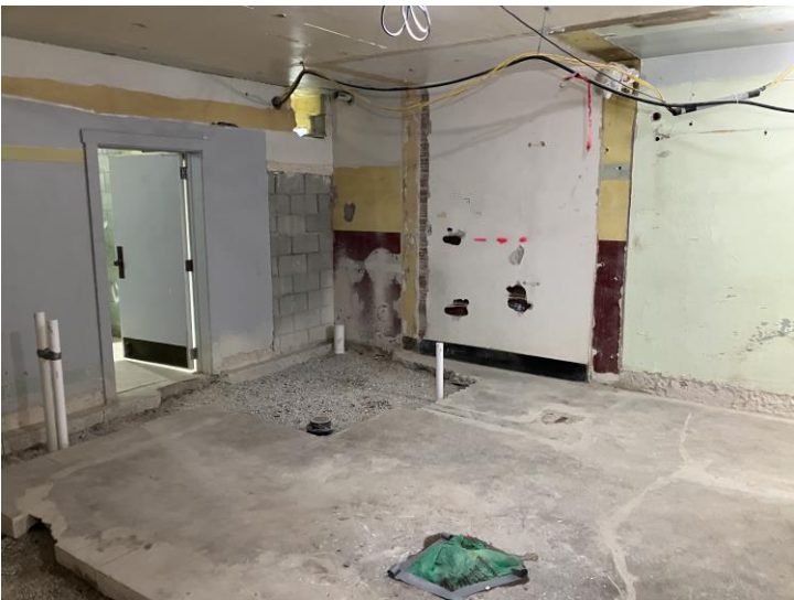
Backfill of underground plumbing after passed inspection
