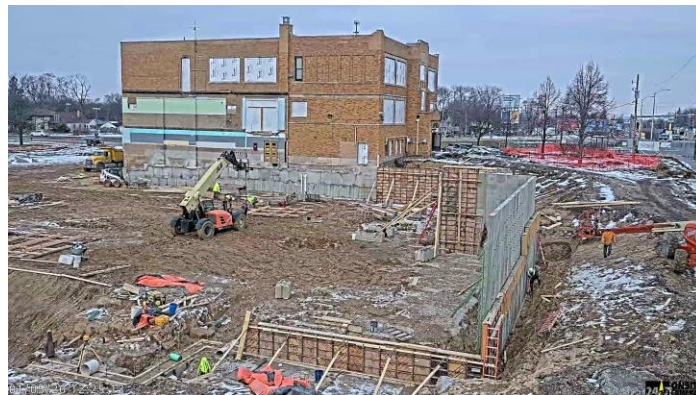
Building B southeast wall poured
