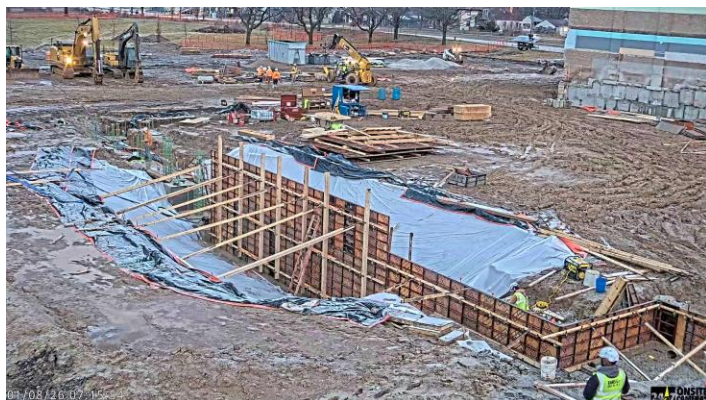
Southside of Building B wall forming
