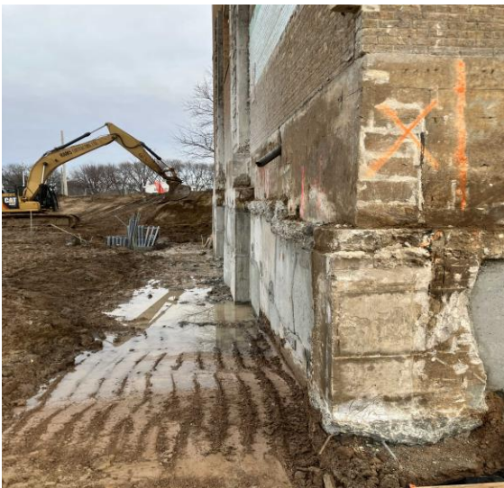
Underpinning building A west end complete
