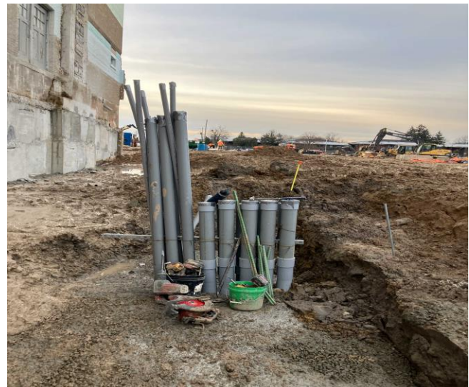
Electrical tubing on westside of building A
