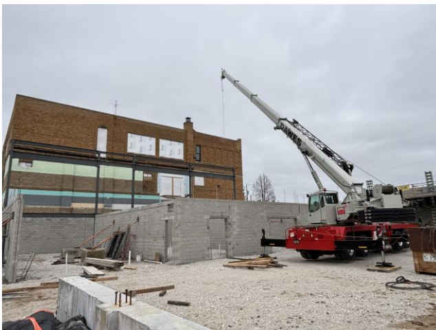
Structural Steel Erection – Area B
