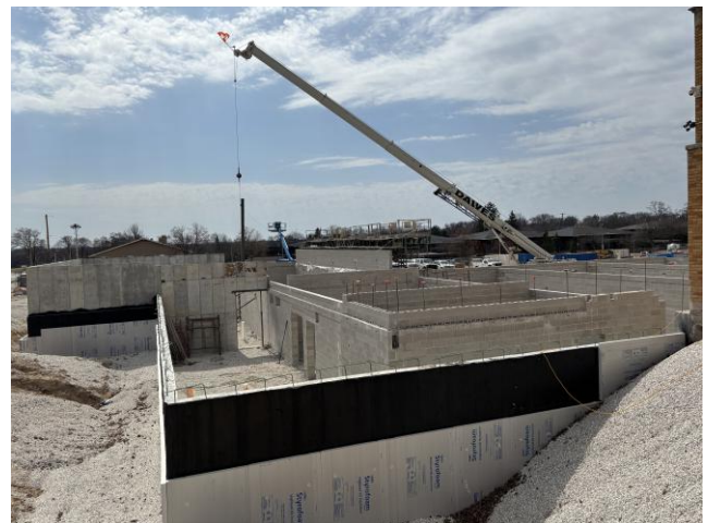
First Structural Steel Column Installed Area B!
