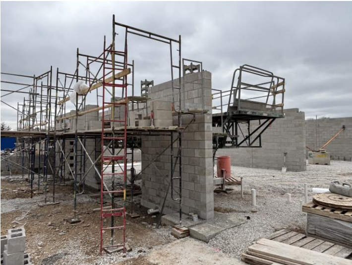
CMU Walls - Vocational Training Rooms Ground Floor Area C
