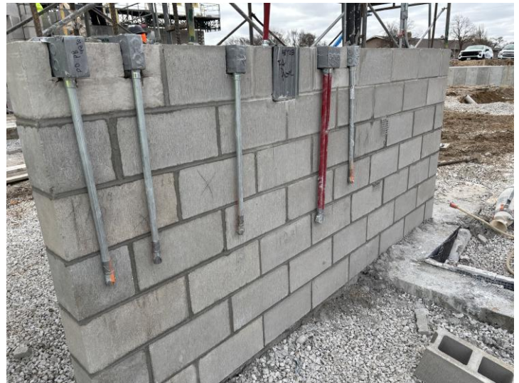
Main Entrance Vestibule C001 CMU In wall electrical rough-in
