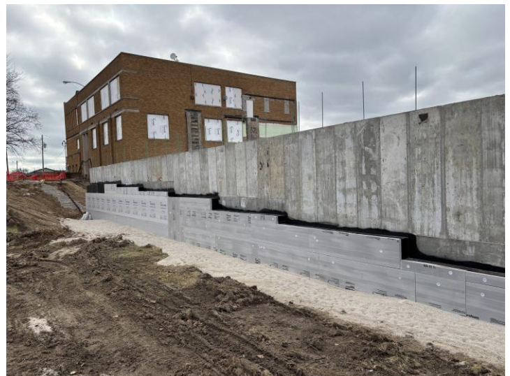
North Wall Area C Gymnasium waterproofing and backfill
