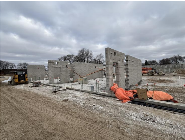
CMU Walls for Vocational Training rooms Ground Floor Area C
