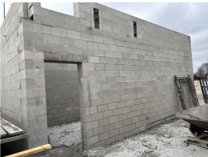
Area C Stairwell #2 CMU install complete for Ground Floor
