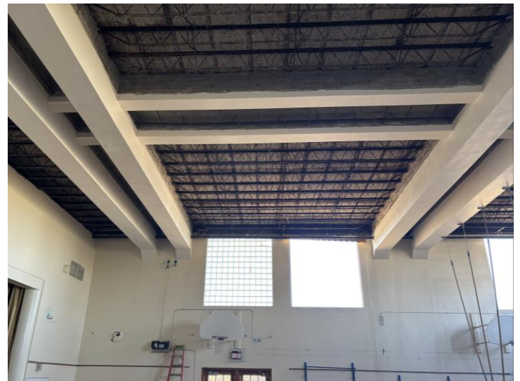
Gymnasium light fixture removal
