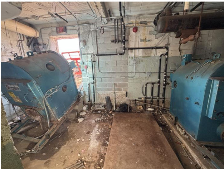
Boiler room demolition
