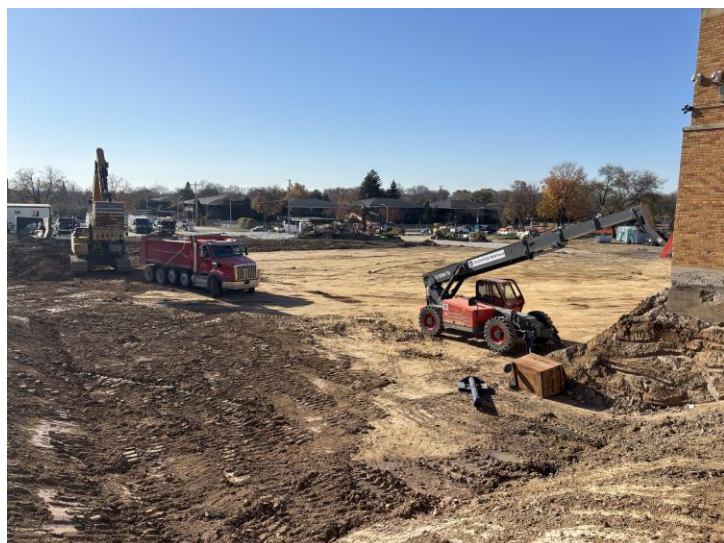
Excavation – areas B & C
