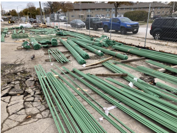
Foundation rebar delivery
