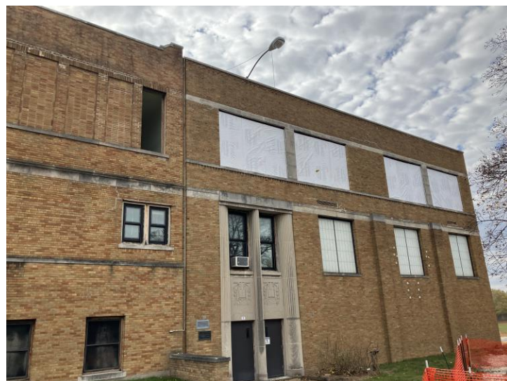
Window removal and temporary enclosures
