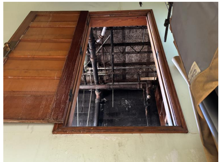
Interior MEP demolition above auditorium stage
