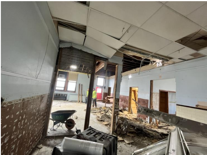
Interior selective demolition – level 3
