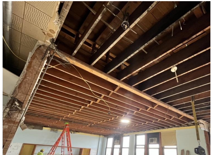
Interior selective demolition – level 3
