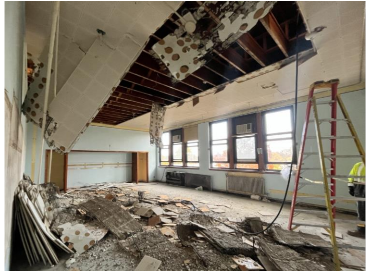
Interior selective demolition – level 3
