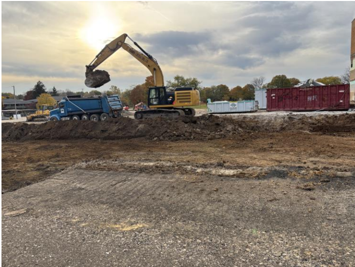
Excavation area B
