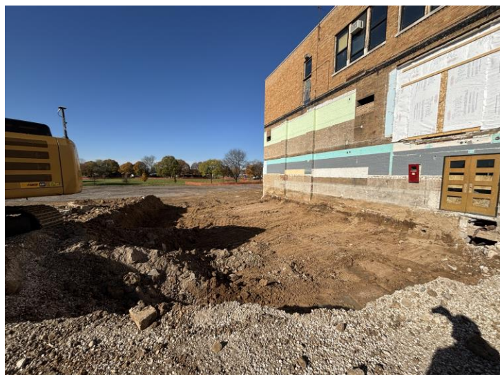
Excavation area B
