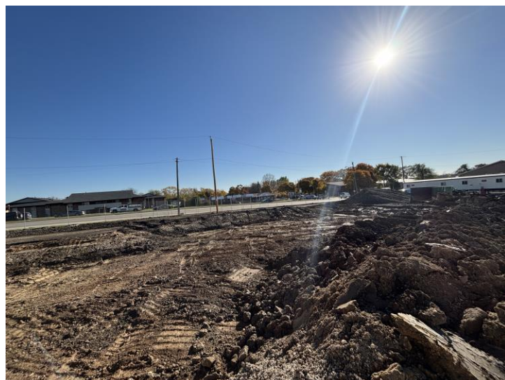
Excavation area B
