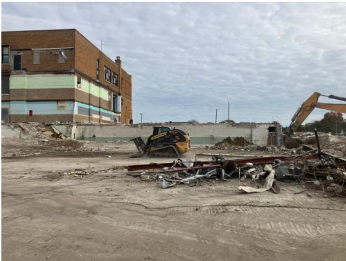
Mass demolition of addition
