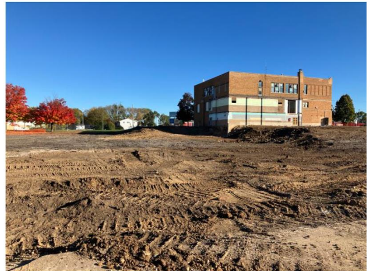
View of existing structure from Southwest
