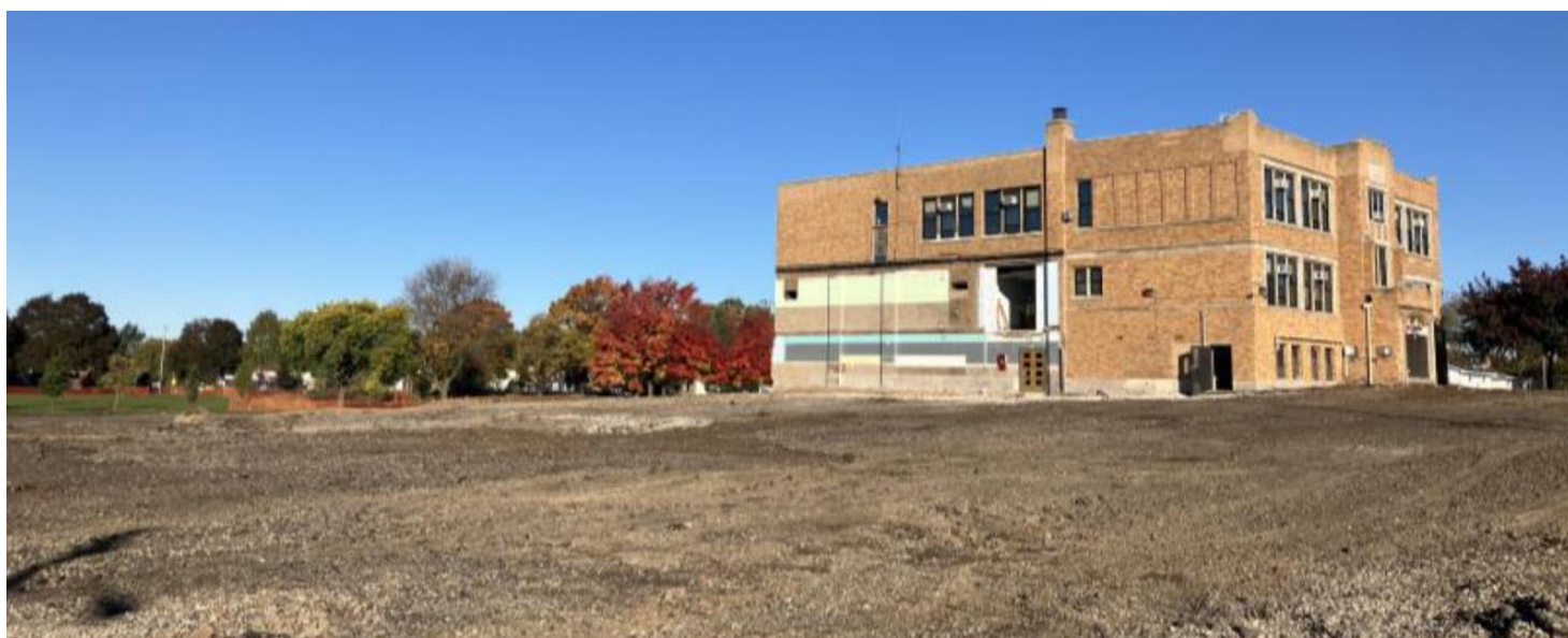
View of existing structure from Southeast
